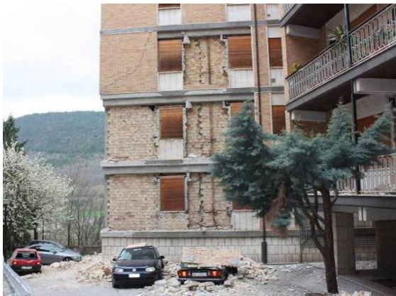
Photographs: Structural and non-structural damage examples on RC buildings after the L'Aquila 2009 earthquake (Photographs by Braga et al., 2011).
