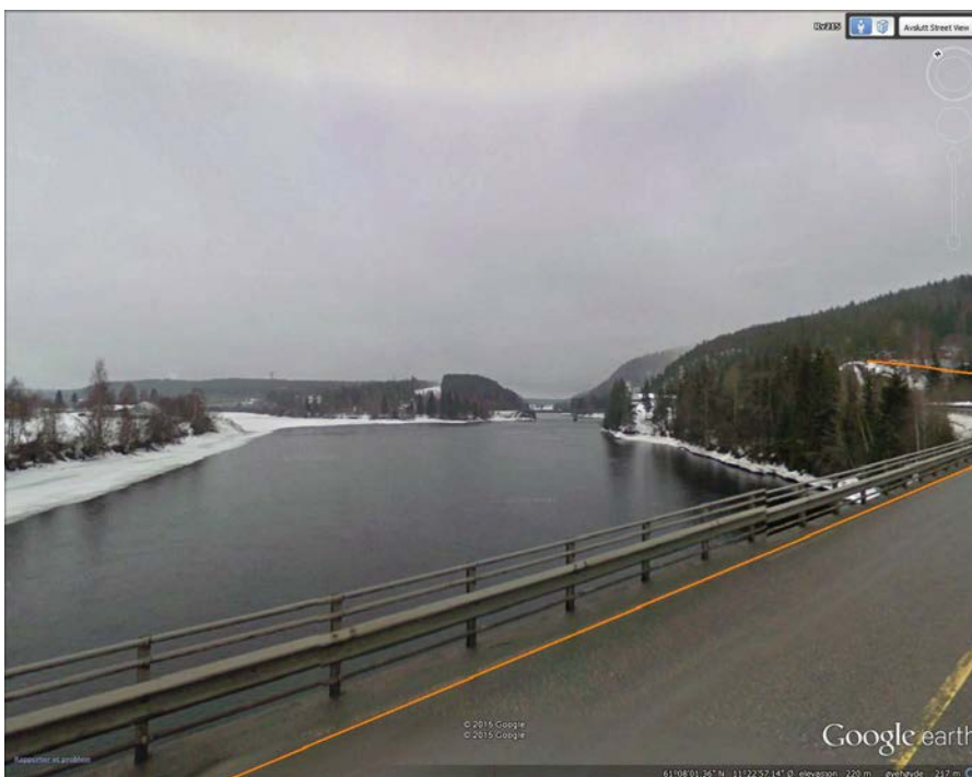
Figure 4.2 Google Earth street view in the direction of the Tx at Rena
