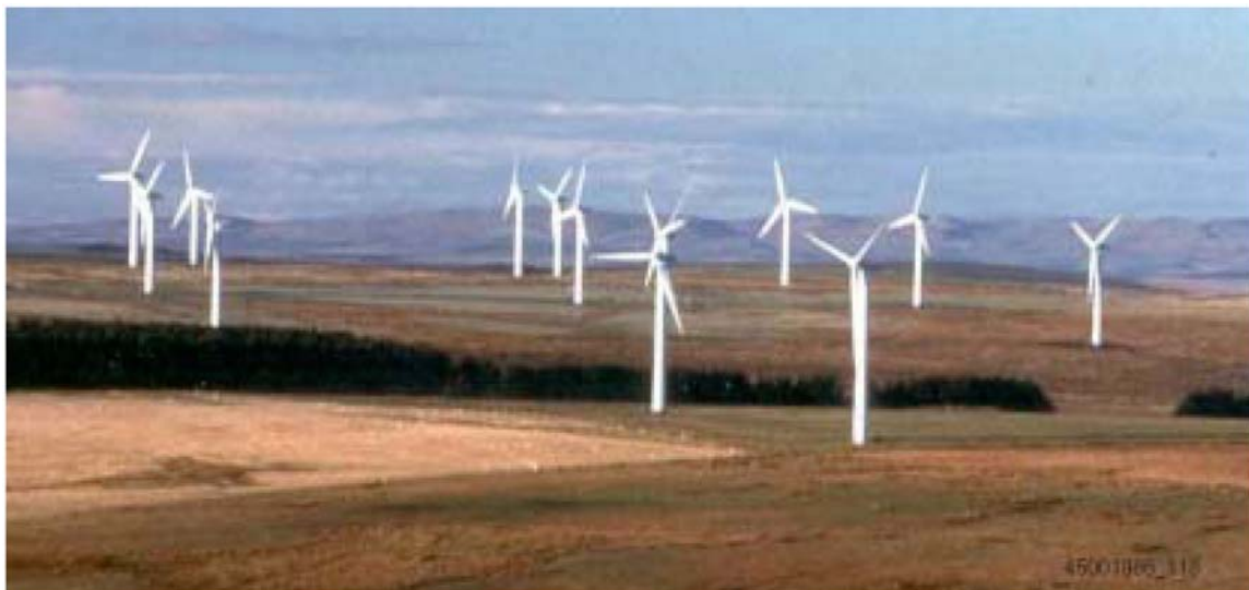
A Typical Wind Farm Cluster - Dun Law Wind Farm Photo courtesy of Renewable Energy Systems
