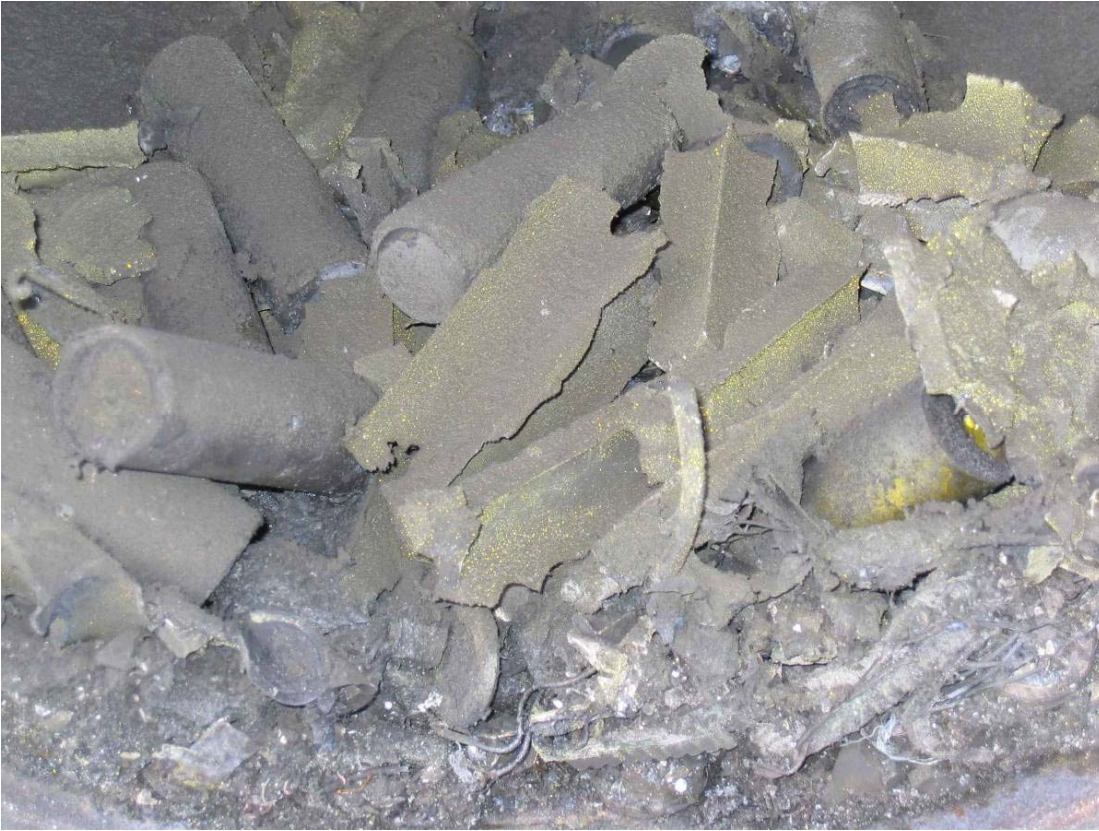
Figure 5.28 The cell modules after the explosion. Note concave bulge in the cell bottom. Note also the yellow powder on the cells (sulphur?)
