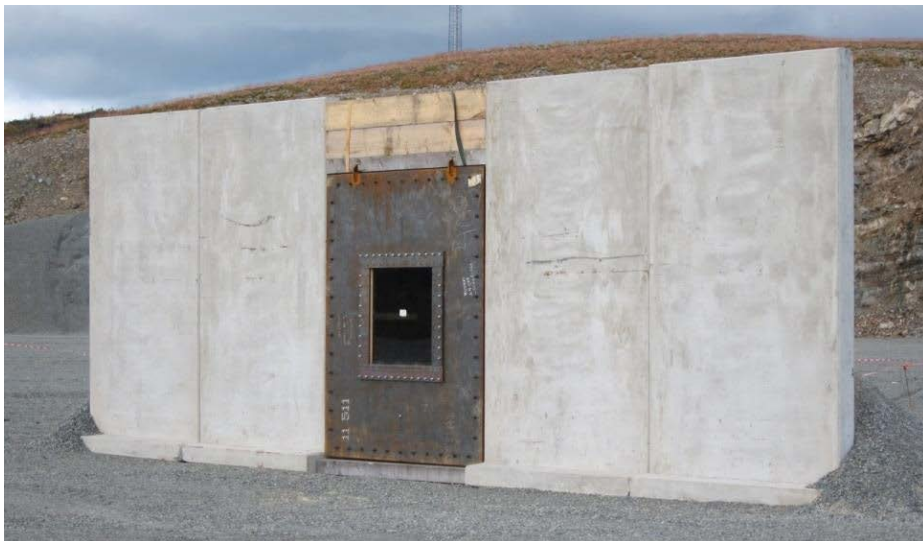
Figure 5.7 Test structure with chamber and concrete walls [33]
