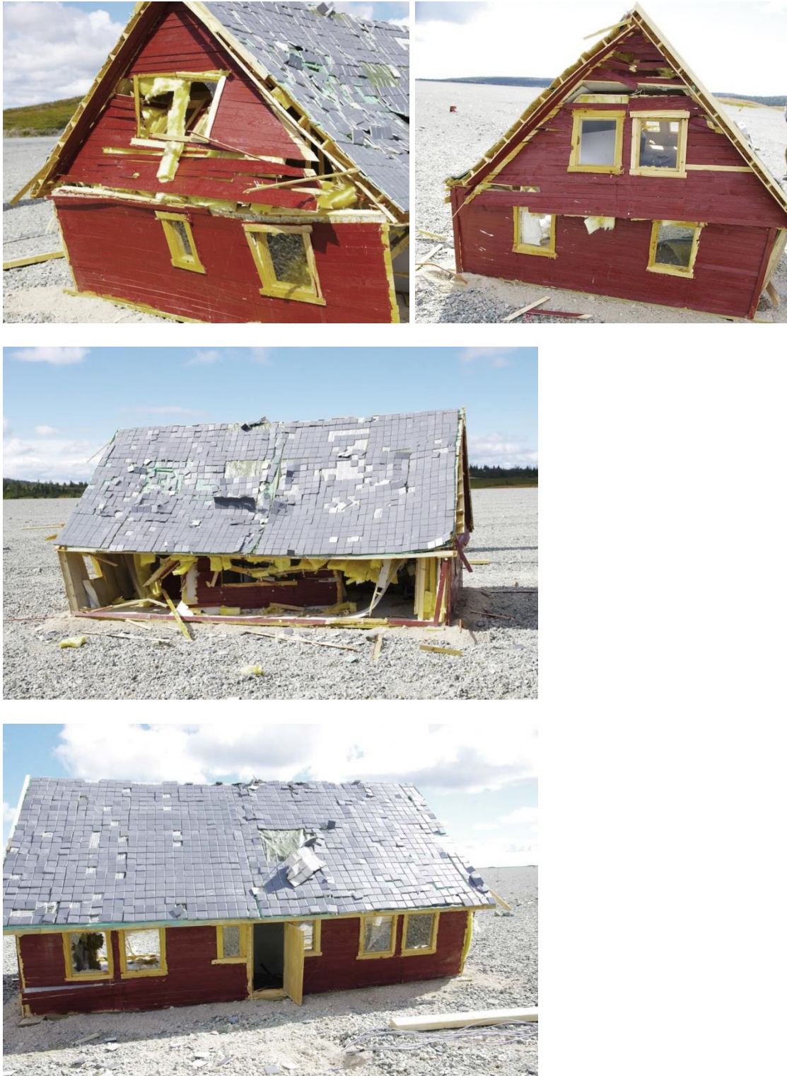
Figure 5.11 Lykkebo in scale 1:5 after detonation of 350 kg Texit 35 m from the house
