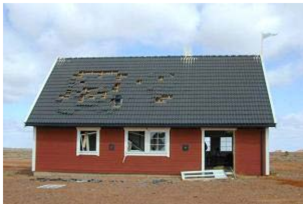
Figure 5.5 Front wall of Lykkebo after the five tonne trial [29]
