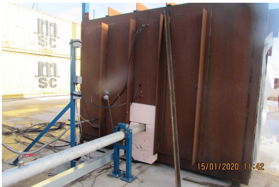
Figure 3.13 Sealing to make TCS tight. Blue stand with white boxes to the left shows the thermocouples and oxygen sensors.
