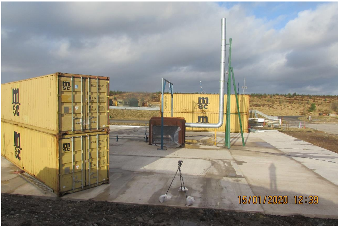
Figure 3.1 Test facility with enclosure connected to ventilation mast for the closed room leakage tests. The tripod in front was for the camera filming the experiments.
