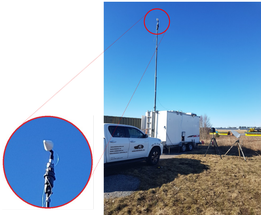
Figure 4.6 Antenna installation on a 10-meter high mast.
