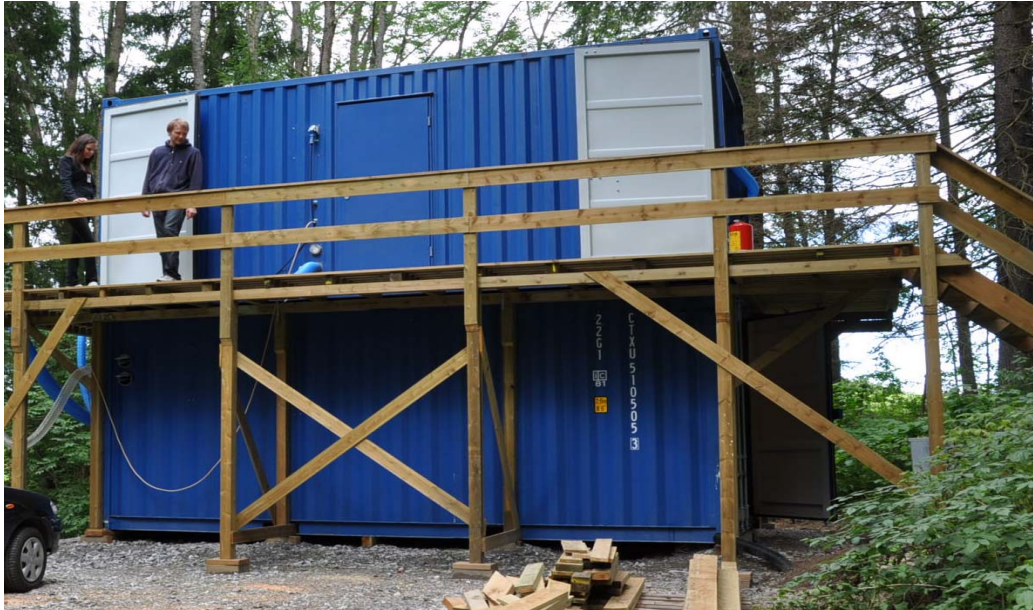
Figure 3.4 FFI semi-closed chamber release system with release container placed on top of service container
