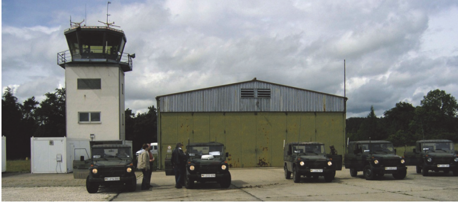
Figure 7.2 Tower where the gateway node between the convoy and the rest of the CoNSIS network was placed. All radio types used by the convoy were also installed in this tower.
